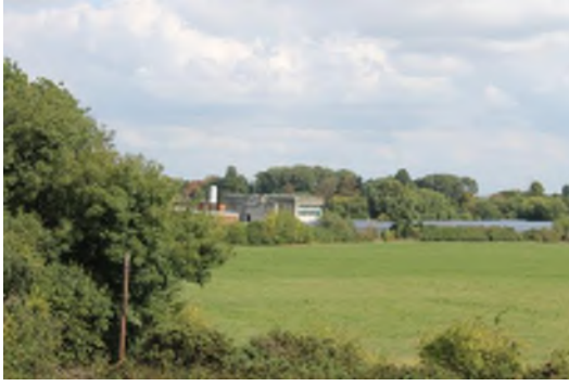
View towards Chertsey Water Treatment Works
