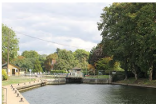
View to the lock.
