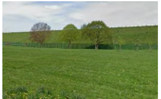
Queen Mary Reservoir embankment
