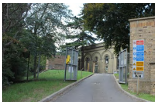
Desborough Island Water Treatment Works
