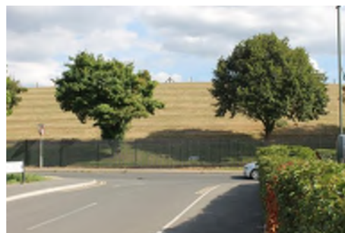
Embankment of Knight Reservoir
