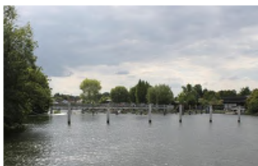
Weir and lock infrastructure
