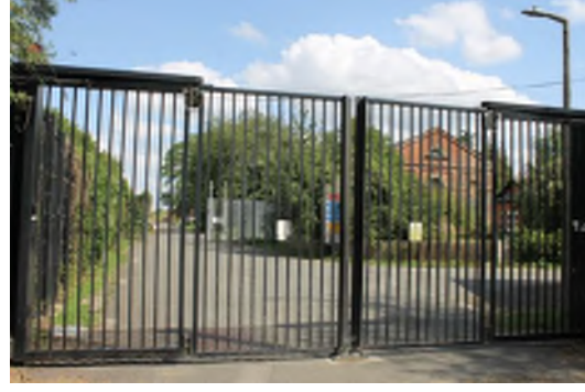
Chertsey Water Treatment Works
