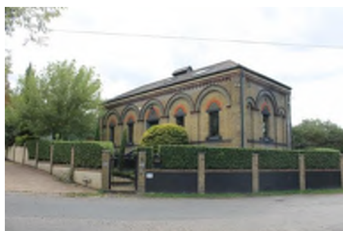
Pump House – now a residential property
