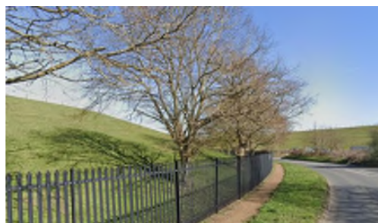
Reservoir embankments – Knight (left) and Queen Elizabeth II Storage (right)
