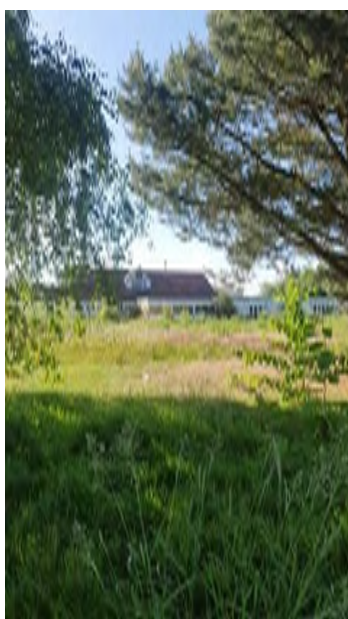
View of disused clubhouse
