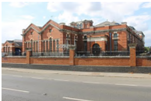
Walton Advanced Water Treatment Works
