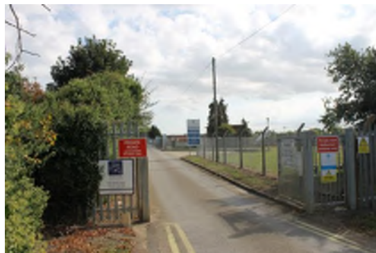
Windsor Sewage Treatment Works
