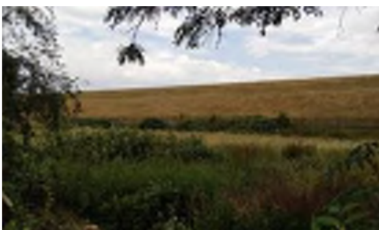
Embankment of Wraysbury Reservoir
