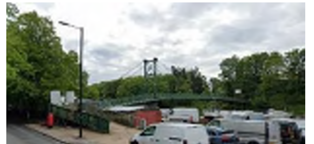
Ornate footbridge to Platt's Eyot
