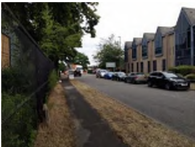
View within character area showing boundary treatments and commercial units
