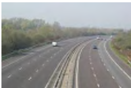
M3 from footbridge
