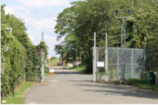
Raised bank of the reservoir visible in the distance
