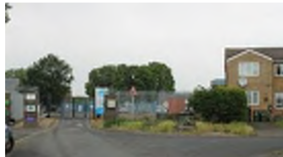
Entrance to Esher Sewage Treatment Works
